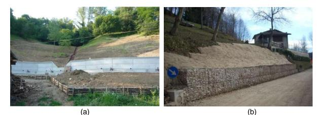
Figure 3. Examples of wall in Vicenza Province: a cantilever tied-back wall realized at Lusiana (a); a gabion wall in Valli del Pasubio (b).
