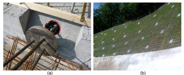
Figure 6. Anchor connection plate during installation (a); a soil nailing with flexible face in Vicenza (b).
